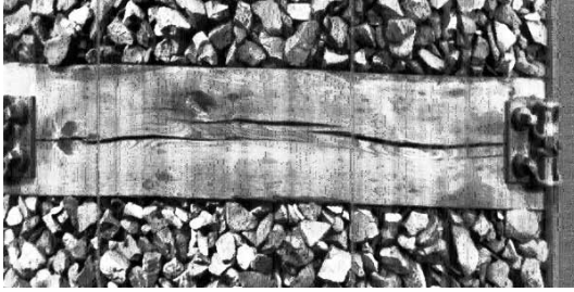
Figure 3: Image after histogram equalization and illumination homogenization
