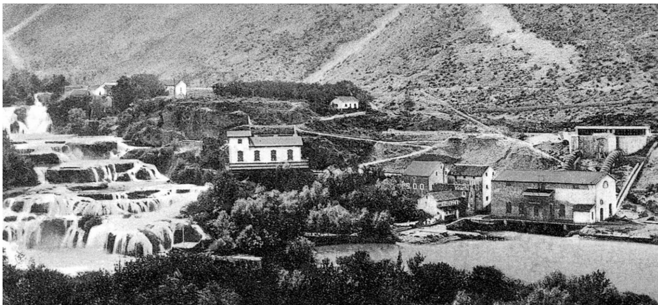
Fig. 4. Hydro plant Jaruga 1 in 1904 (taken from [12])
