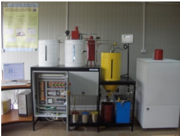
Fig. 1. Wastewater treatment pilot plant from “Dunarea de Jos” University of Galati
