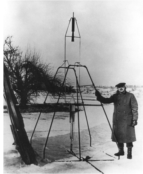
Fig. 3: Goddard and his liquid fuel rocket. Note that the gas exhaust at the top is over the liquid fuel and oxygen tanks. This design is no more stable than having the exhaust at the bottom. (NASA, Public Domain)
