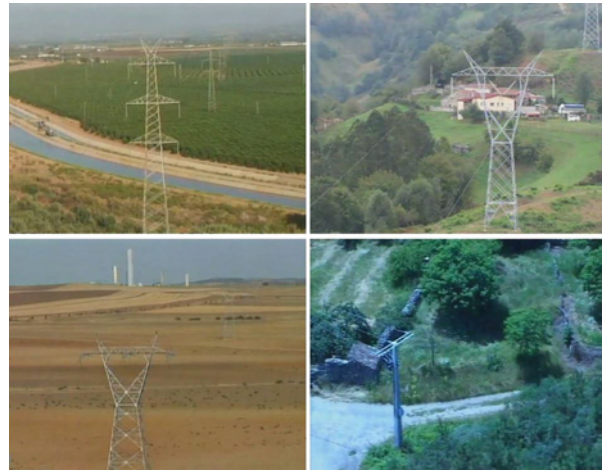
Fig. 1. Power line inspection. The inspection of power line infrastructures is a very challenging task for computer vision algorithms, due to the large variety of backgrounds and types of tower.
